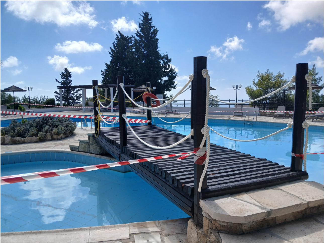
The bridge has been fixed and painted
